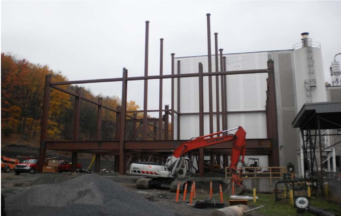
Erection of structural steel supports
