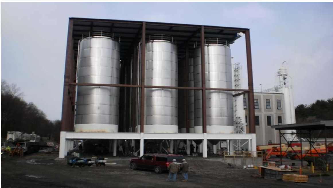
Completed structural support for fermentation tanks for Yuengling brewery expansion in Pottsville, PA
